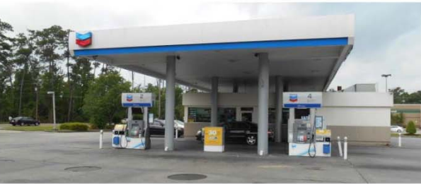
Chevron Gas Station
